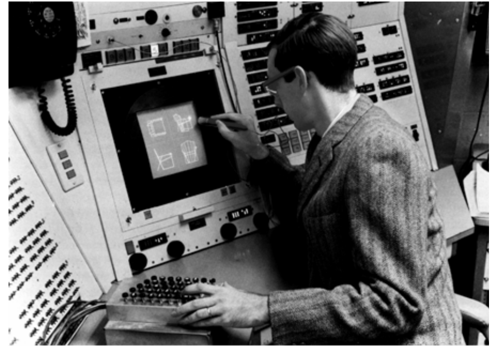
Sketchpad in 1963. Note use of a CRT monitor, light pen, and function-key panel.
